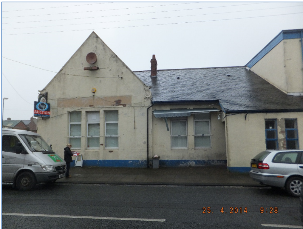
Photograph 1 Property exterior (eastern elevation)
